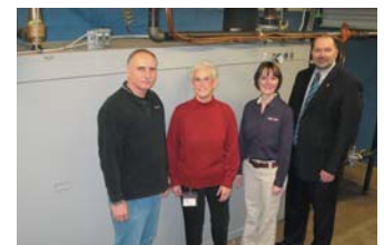
Pictured with the new boiler are (left to right) KSI's Shawn Bowman, Discover Bank's Sherry Berman and Amy Walls, and KSI CEO, B. Craig Crouch.
